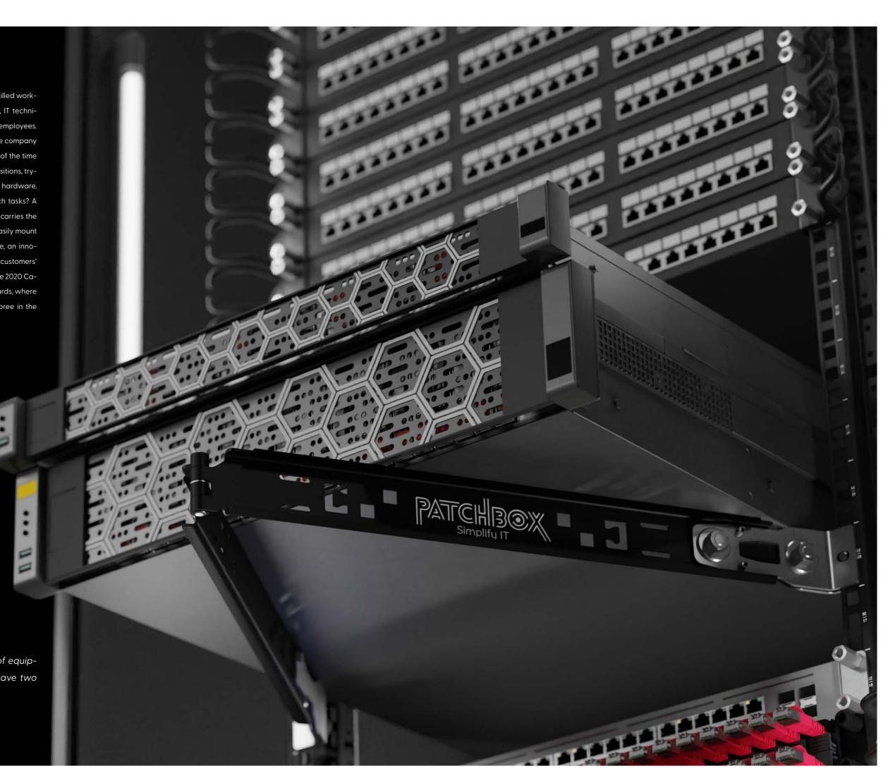
The Setup.exe can carry up to 50kg (110lbs), holding onto expensive hardware until it is securely mounted. It can be mounted facing inwards to help with guiding hardware easily into the network rack, or it can be faced outwards of the cabinet. By doing that, the rubberized side on top acts as a shelf to carry your laptop safely. The sides of the Setup.exe provide you with holes to mount velcro, cable ties and spare cage nuts.
